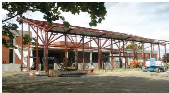
A recent look at the progress on the campus' newest addition
